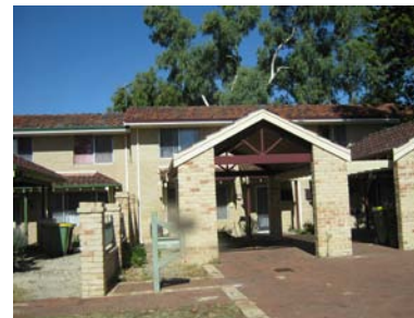
The townhouses with new carports show signs that some tenants are prepared to invest time into maintaining / improving presentation
