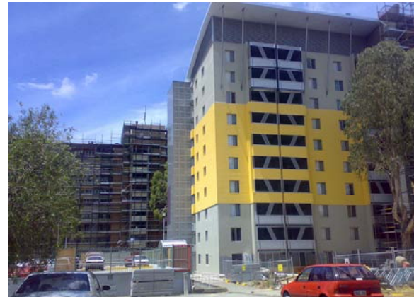
Figure 7. Recent photo of the extend of renovations
