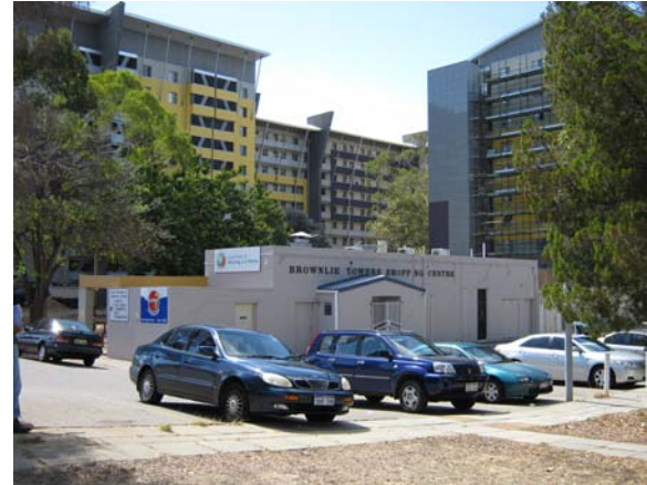
Figure 6. Recent photo of the extend of renovations
